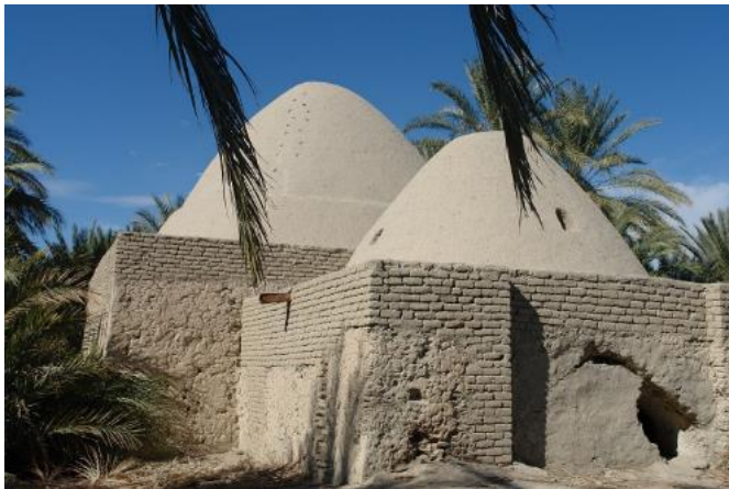
Figure 21. Outside view of tomb No. 4, after restoration, (2010), (photo:M. Keyhanpoor)
