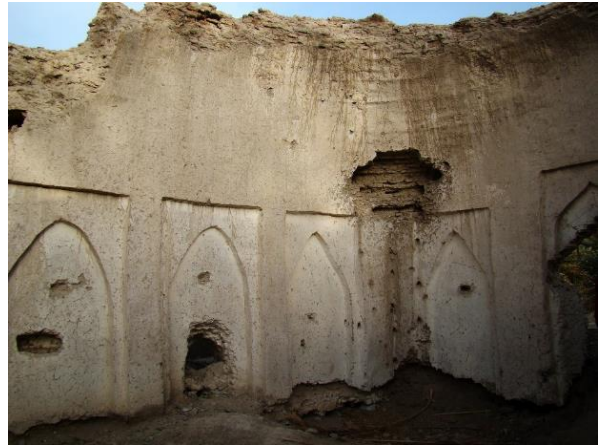
Figure 18. tomb No. 3, General inside view-before restoration (Arcades & Squinch), (2011), (photo:M. Keyhanpoor)
