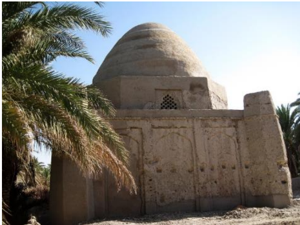
Figure 20. Tomb No. 1 After restoration, outside view, (2010-11), (photo:M. Keyhanpoor)
